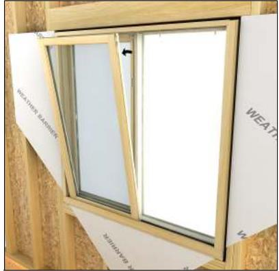
2. Tilt and remove the sash.
