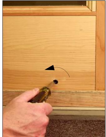
by turning a flathead screwdriver in the adjustment holes at the base of your operator panel. If the gap appears wider at the bottom, first adjust the roller closest to the frame upward or the roller near the stationary panel downward until the panel sits level on the track.
