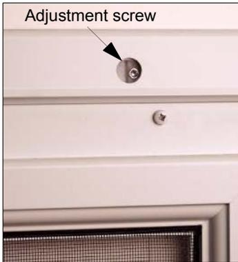
Screen adjustment is possible by loosening or tightening the adjustment screw found in the roller bar assembly. Slide screen panel so that adjustment screw lines up with access hole. Turn the adjustment screw(s) counterclockwise or clockwise. An even reveal should be achieved along the entire height of the jamb. For detailed instructions on how to install the screen, see our [installation instructions](#) or go to our website [www.marvin.com](http://www.marvin.com).
